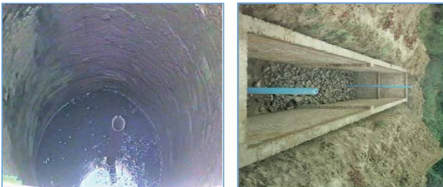
Figure 8. Artificial groundwater recharge structure at President's estate.
