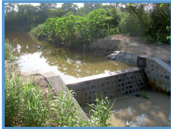
Figure 3. Check dam for surface water harvesting.
