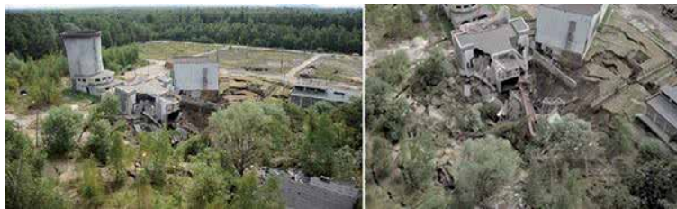
Figure 1. Sinkhole and remains of shaft V, Szczygłowice colliery [6].
