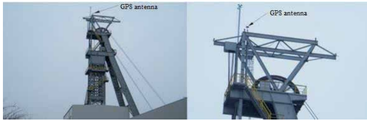
Figure 6. Head frame of S1.2 shaft, LW Bogdanka coalier.
