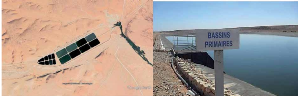
Figure 2. Ghardaia wastewater treatment plant.
