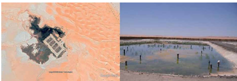
Figure 13. N'Goussa wastewater treatment plant.
