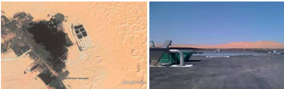
Figure 8. Sidi khouild wastewater treatment plant.
