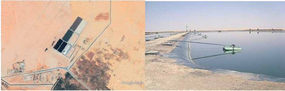
Figure 6. Ouargla wastewater treatment plant.
