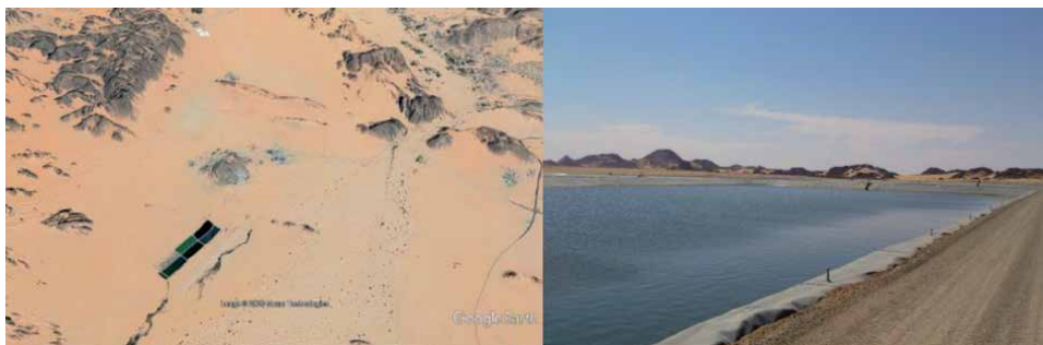
Figure 4. Djanet wastewater treatment plant.
