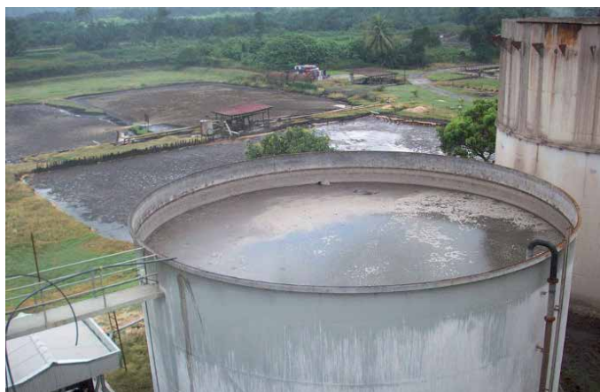
Figure 5. Typical open digester tank.
