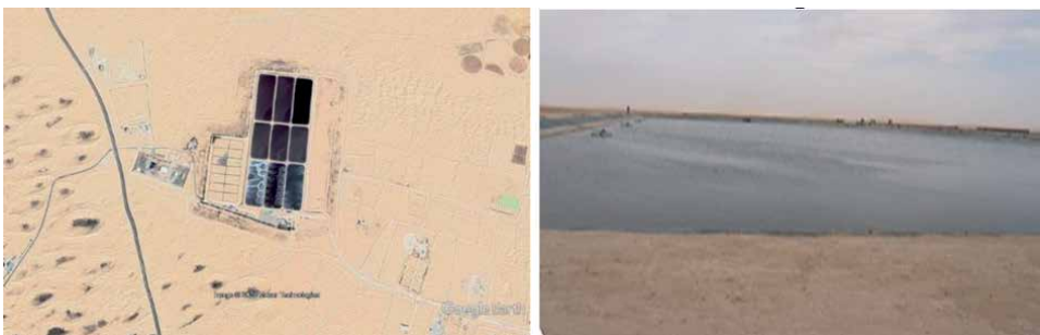
Figure 9. Kouinin wastewater treatment plant.
