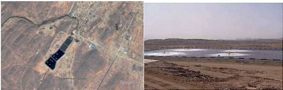
Figure 7. Tamannasset wastewater treatment plant.
