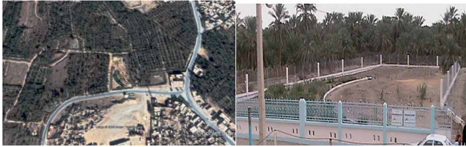
Figure 12. Temacine wastewater treatment plant.
