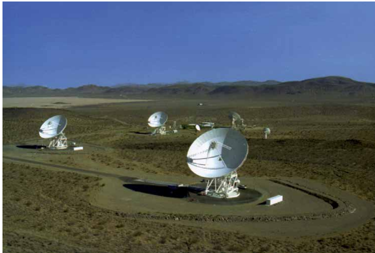
Figure 20. Parabolic reflector antennas at The NASA Deep Space Network Goldstone Ground Station Complex (image courtesy of NASA).
