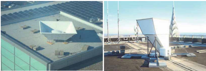
Figure 1. A radar wind profiler (left) mounted on the liberty science center and a sodar wind profiler (right) mounted on a NYC high rise [8].
