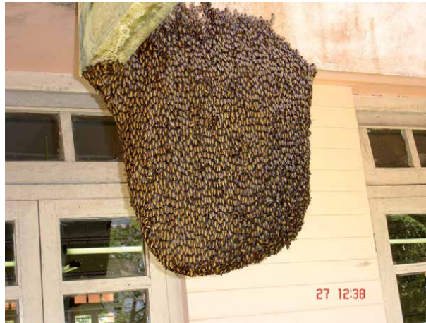
Figure 14. Apis dorsata – A Rockbee colony on building corner of BSI at Port Blair (2014).
