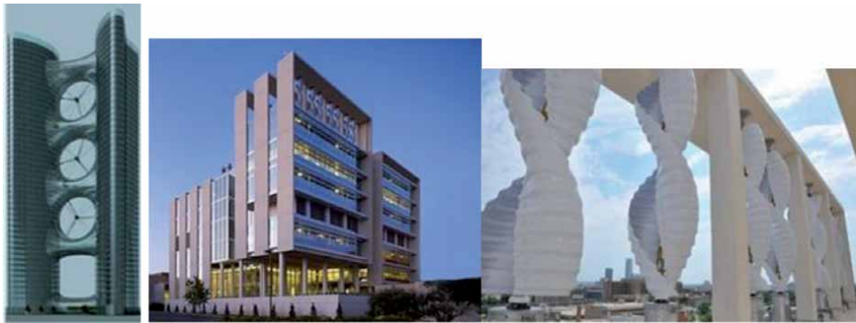
Figure 10. Wind turbines integrated into the building [20, 21].
