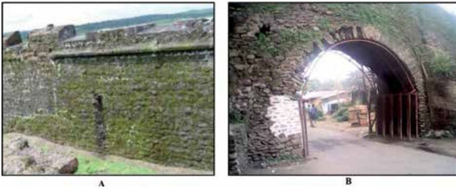
Figure 11. Biological growth at Fort San Lorenzo (Panama); source and Fasil Ghebbi [source; Eskinder Desta]. A. Biological growth at Fort San Lorenzo (Panama). B. Biological growth at Fasil Ghebbi.
