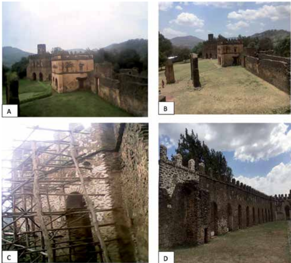
Figure 12. Some selected spots inside the royal palace before and after restoration. (A and C): in 2015; (B and D): in 2019 [source; Eskinder Desta].
