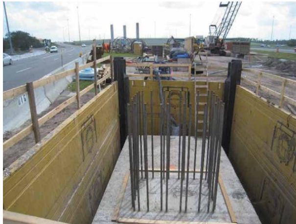
Figure 3. Bridge footing for monitoring in Orlando, Florida.
