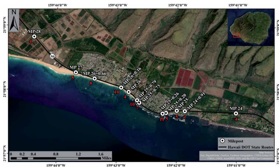
Figure 21. Ocean Hazards Classification Scheme (OHCS) ranking for Kauai West Kauai (W) MP 24 to 28. The OHCS consists of five variables: (i) sea level rise 1905–2050, (ii) maximum annually recurring significant wave height 2010–2018, (iii) shoreline change 2008–2100 and CRESI Armoring, (iv) historical and hypothetical tsunami, and (v) Category 1,2,3,4 hypothetical storm surge. Rankings of ocean hazard increase from 1 to a theoretical maximum of 100.
