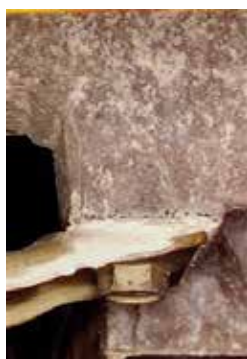
Fig. 4. Magnesium alloy casting fastened to a steel bracket using a coated steel bolt. The interface between the steel bracket and the magnesium casting surface is prone to galvanic corrosion.
