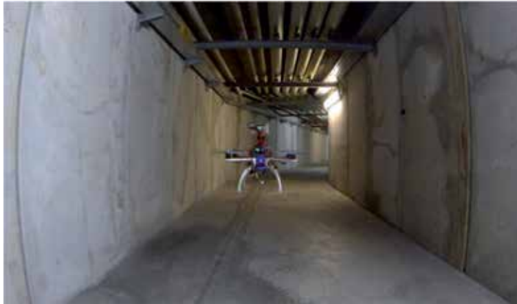
Figure 11. Tunnel inspection performed by the UAV during the test of system validation.
