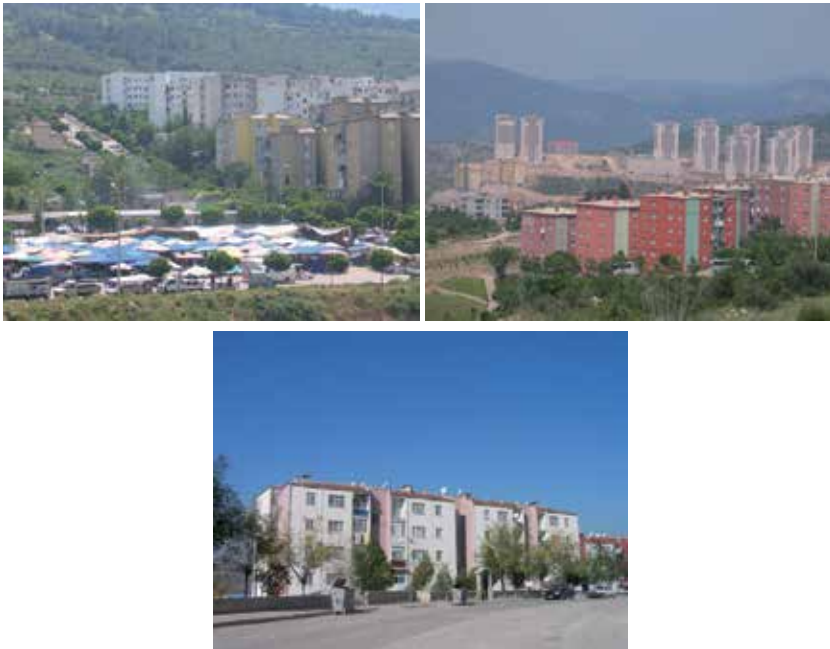
Fig. 6. Examples of social housing blocks in Bursa (A.I.Çahantimur archive)
