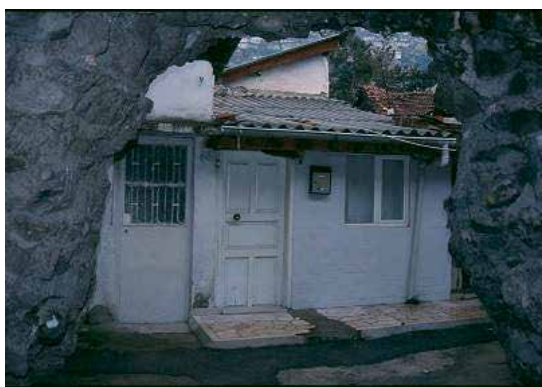
Fig. 15. A house between the historic city walls (A.I.Çahantimur archive)
