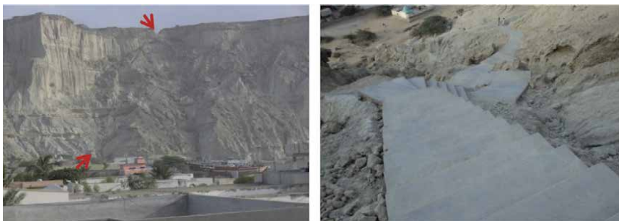
Figure 2. Pedestrian tsunami evacuation route at Gwadar City, Baluchistan Province. (Left) Red arrows show starting and ending point of the evacuation route. (Right) Tsunami evacuation route, more than 600 steps of a stairs designed with landing at several points to facilitate pedestrian evacuation leading to the proposed evacuation site at the top of the Koh-e-Batil (a 450 high mountain) by the district disaster management authority Gwadar. Photo by Ghazala Naeem.
