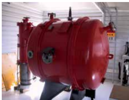
Fig. 4. Photograph of the vacuum chamber and diffusion pump for high vacuum
