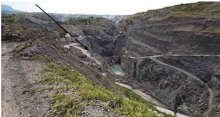
Figure 11. Free rock slide and falling site in Şırnak Asphaltite open quarry No 2, free slide over excavation area, 1/1000.
