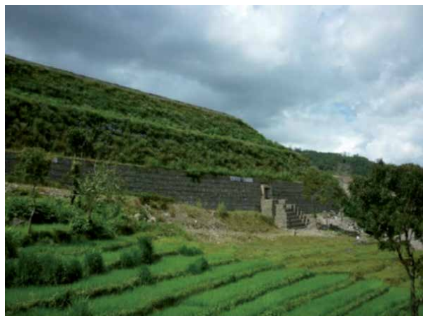
Figure 6. Slope face completely covered with vegetation few months after installation (after [7]).
