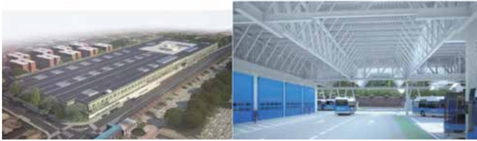
Figure 14. New 100% electric operation Centre La Elipa (project finished).
