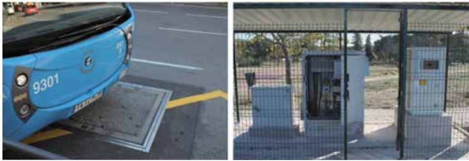
Figure 10. Bus charging by induction and necessary installations.
