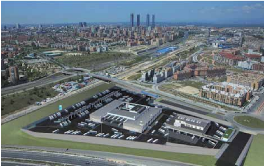
Figure 13. View on the Sanchinarro operation Centre built in 2010.
