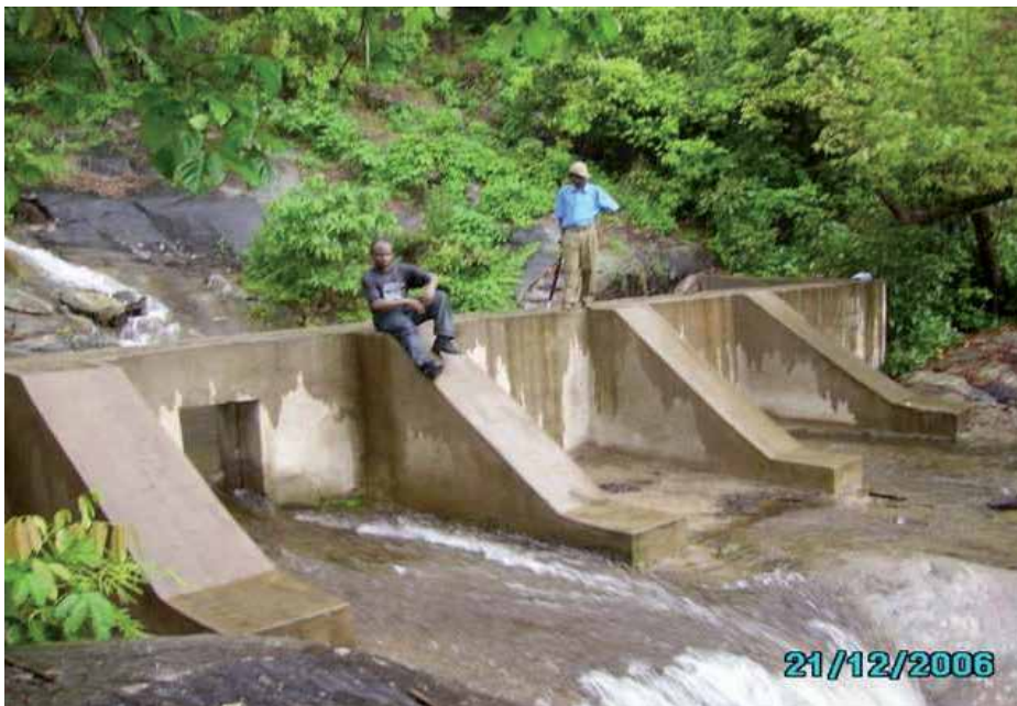
Fig. 3. Water falls for mini-hydro power at Chita-Kilombero
