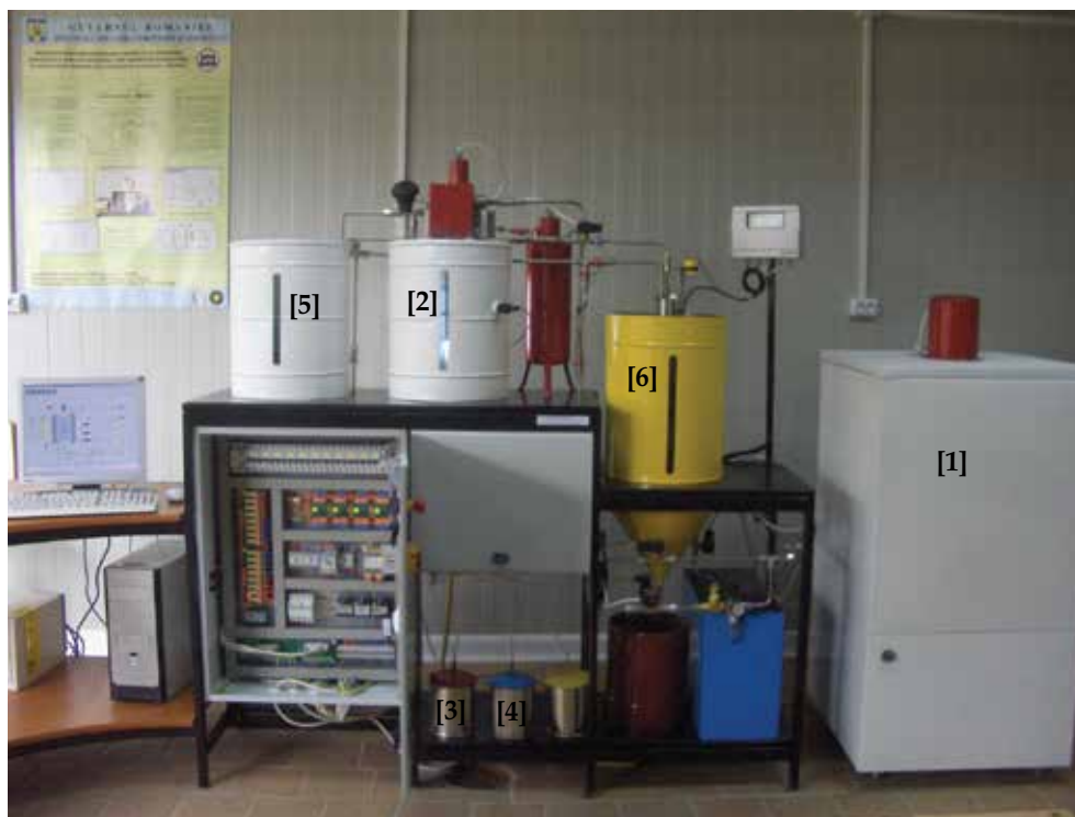
Fig. 1. Wastewater treatment pilot plant
