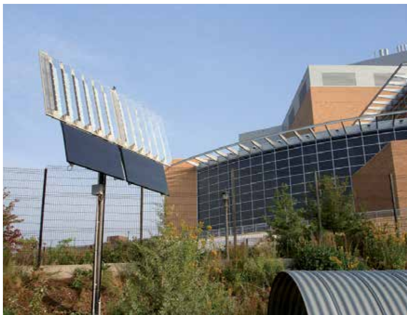
Fig. 9. Dual-axis solar tracking LCPV design with 3M brand Cool Mirror (Minnesota Science Museum).
