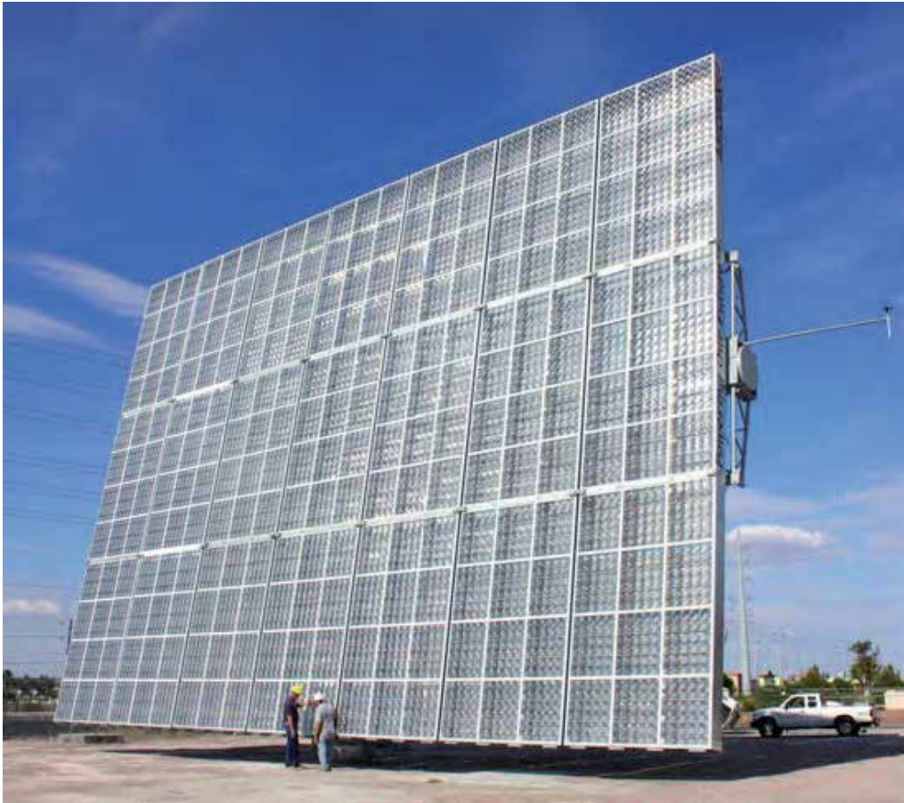
Fig. 4. The Amonix 7700 60 kWac System uses high efficiency multijunction solar cells.
