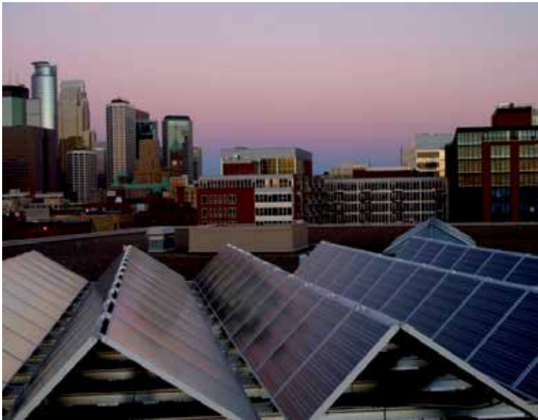
Fig. 4. Non-tracking LCPV design with 3M Cool Mirror (photo courtesy of Ray Colby with Sundial Solar).
