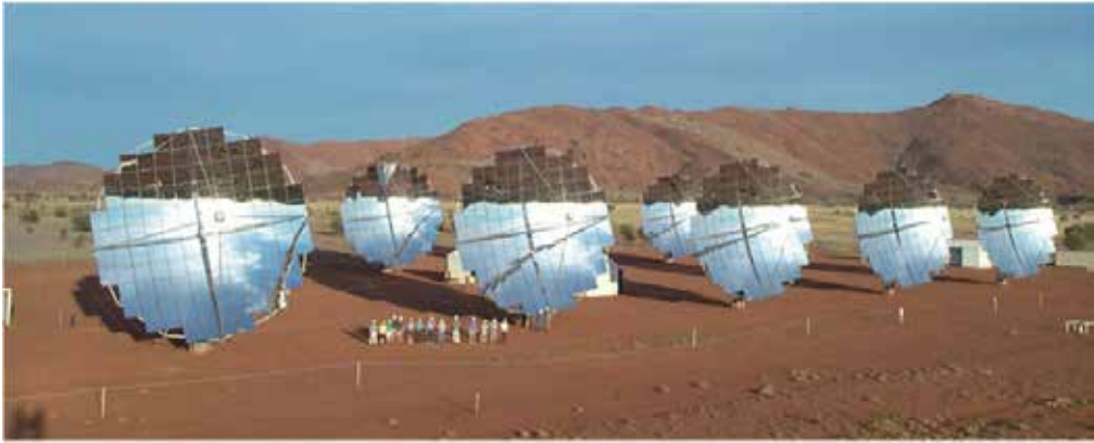
Fig. 3. Several 25-kW CPV systems built by Solar Systems in Hawthorn, Australia, and installed on aboriginal land. These systems use mirrors for concentrating sunlight onto silicon solar cells---see www.solarsystems.com.au The people in the foreground give an idea of the system's size (photo by R. McConnell).
