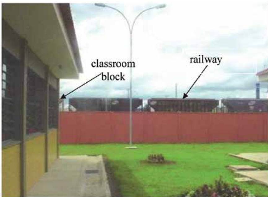
Fig. 8. Classroom C6 and the railroad traffic
