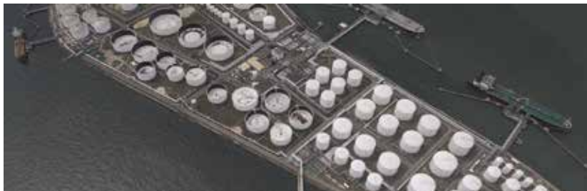
Figure 2. Typical onshore tank farm facility [2].
