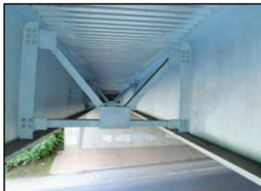
Figure 4. K-type cross brace on Middlebrook Bridge.
