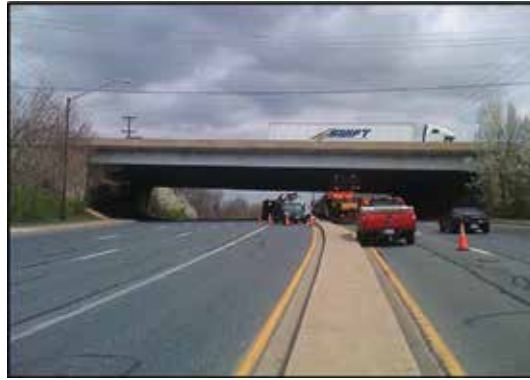
Figure 3. Maryland bridge carrying I-270 over Middlebrook Road.
