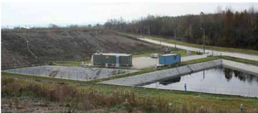
Figure 6. The treatment plant based on the reverse osmosis process (source: [18]).
