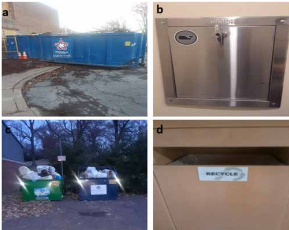
Figure 3. (a) Giant silo bin used to collect and convey building waste at a building renovation site. (b) Indoor waste disposal unit installed in a room to collect house hold waste, which will be channeled out into a silo bin placed outside for onward collection and disposal by waste agent at a building facility in Saint Louis USA. (c) Type I (rubbish, e.g., paper) waste collected and sorted for recycling (green silo).
