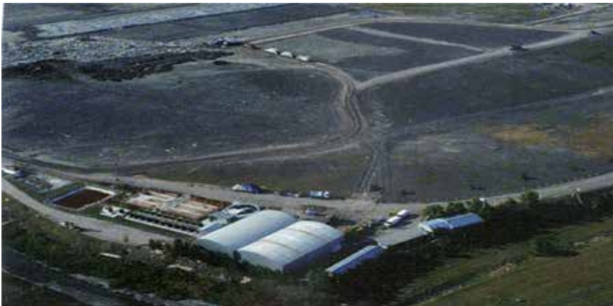
Figure 8. Sanitary landfill Norte III in Buenos Aires (source: [26]).
