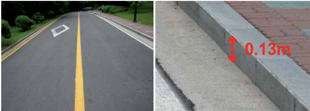
Fig. 3. Road and curb on the road.
