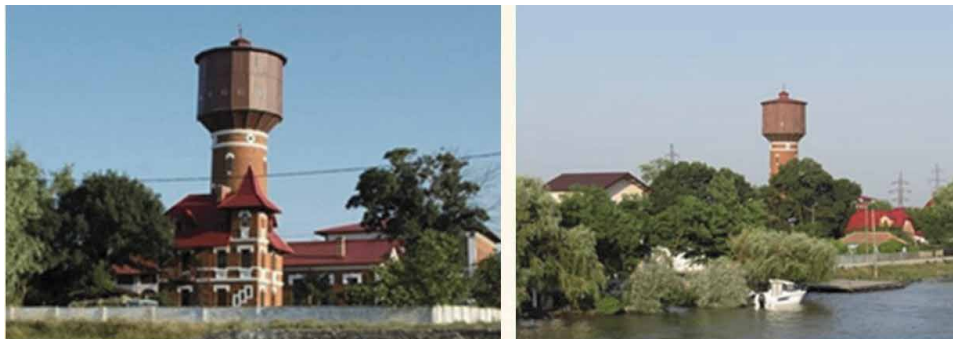
Figure 14. Drinking water treatment plant with the distribution tower in Sulina City.
