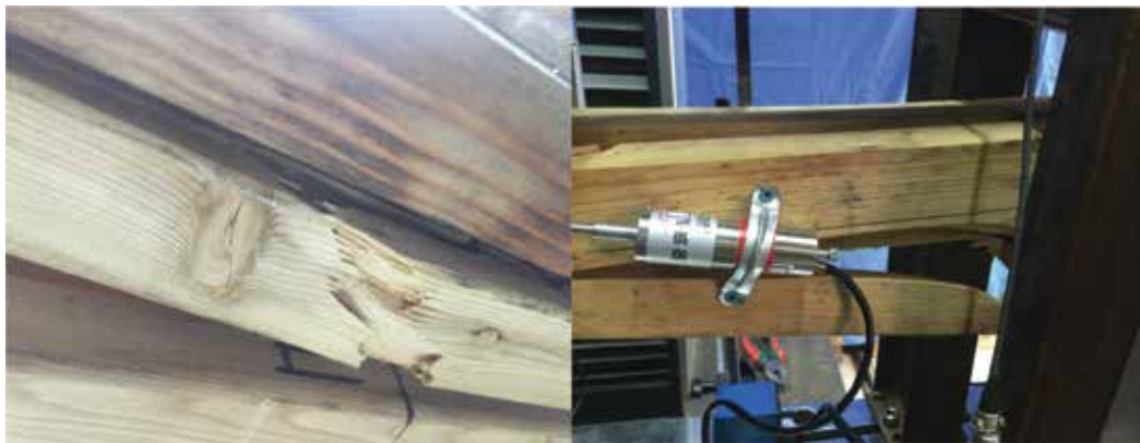
Figure 18. The failure of SPT-G3-16.
