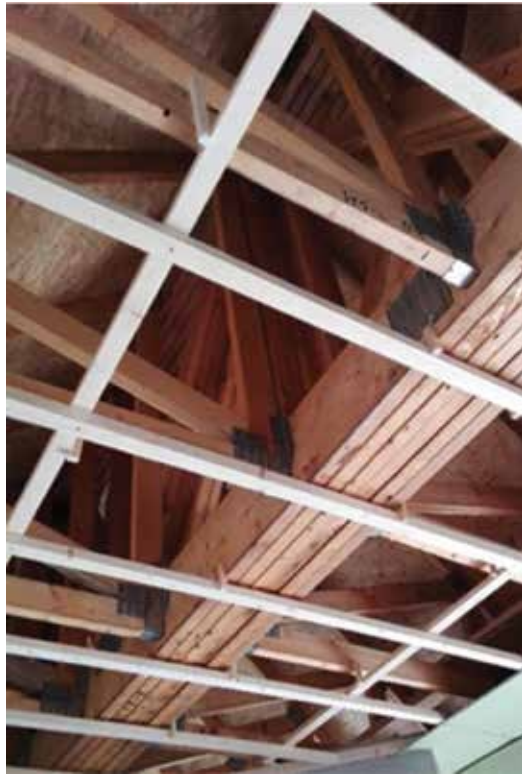
Figure 1. Application of girder truss in building structure.
