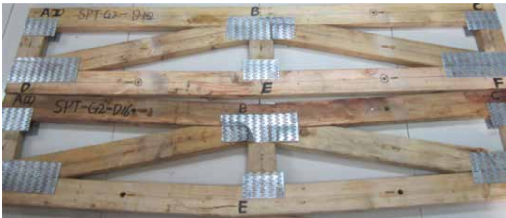
Figure 16. Failure phenomenon of SPT-G2-16.
