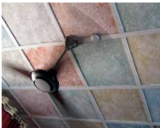
Figure 9. Made-in-Nigeria wood-cement composite ceiling boards after installation. Source: [16].
