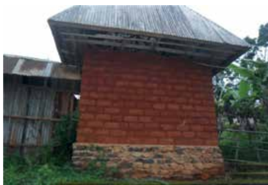
Figure 3. A typical building constructed using clay bricks.
