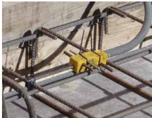
Figure 5. MoniCorr system for linear polarization resistance measurement.
