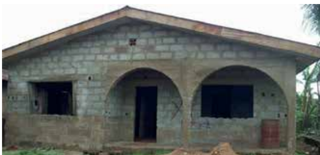
Figure 4. A typical building under construction using concrete hollow blocks.
