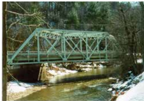
Figure 11. Steel truss bridge on MD 24 over deer creek.
