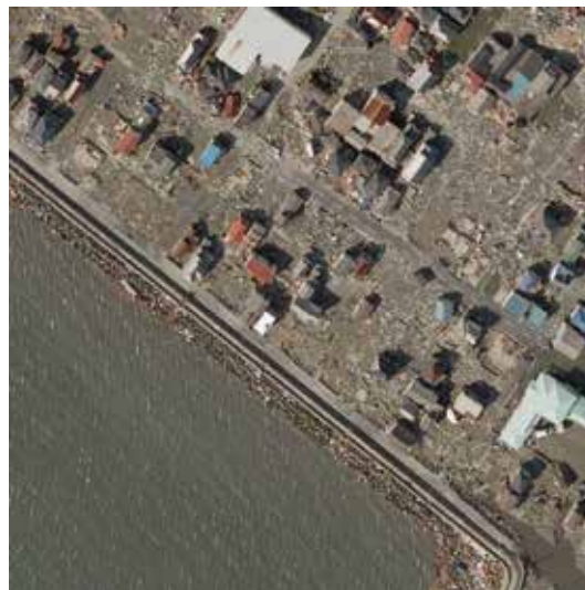
Figure 9. Devastated residential area behind a coastal levee.
