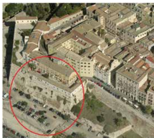
Figure 5. The northwestern sector of the Spanish walls. The circle indicates the survey area.
