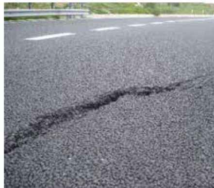
Figure 12. Detail of a fracture in the asphalt at the beginning of the landslide phenomena.
