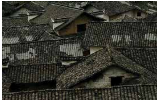
Figure 1. Blue tile roof of Longtan ancient village.
