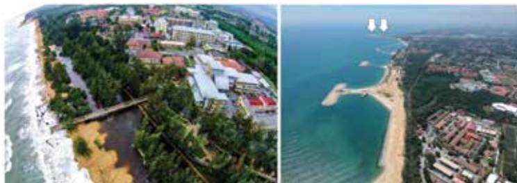
Figure 5. Coastal erosion along the Universiti Malaysia Terengganu (UMT) campus in Kuala Nerus district, north of Kuala Terengganu (left image), and breakwaters constructed to solve erosion along north of Terengganu (right images). White arrows mark extension of airport runway in 2008. Source: Media Kreatif UMT (left image) and Mr. Mokhtar Ishak (right image).
