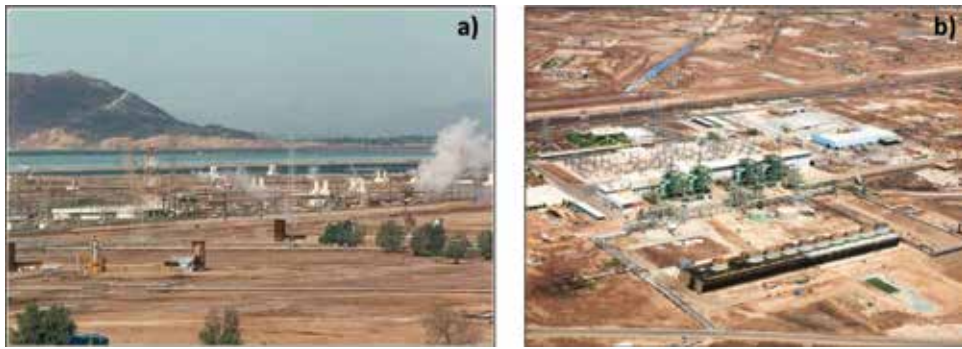
Figure 4. (a) Cerro Prieto Geothermal Power Plant, evaporation pool, and Cerro Prieto Volcano (courtesy of CFE) and (b) Cerro Prieto geothermal power plant (courtesy of CFE).
