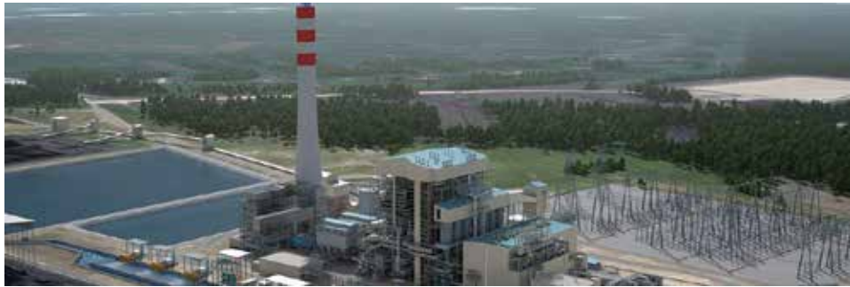
Figure 6. Tanjung bin 4 ultra-supercritical technology. Image: Courtesy of GE POWER.
