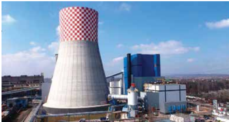
Figure 3. The Łagisza power plant, Poland. Image: Jänttiet al. [16].
