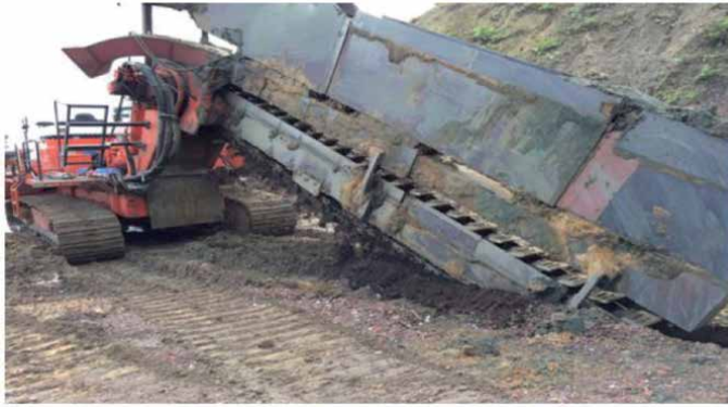
Figure 16. Installation of the deep drainage.
