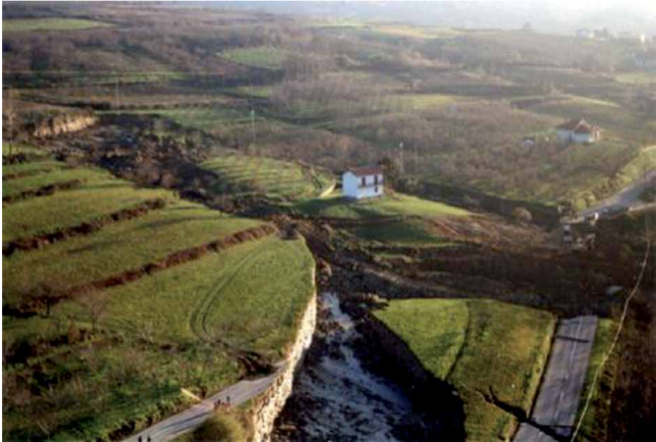
Figure 11. Rock-block slide near Feisoglio town: The mass movement slid about 50–60 m from their original position, destroying a road. The estimated area was about 4.63 ha, while the volume was about 385,000 m 3 . The gray layer surface is evident. The small white house moved together with the rock block nearly undamaged.
