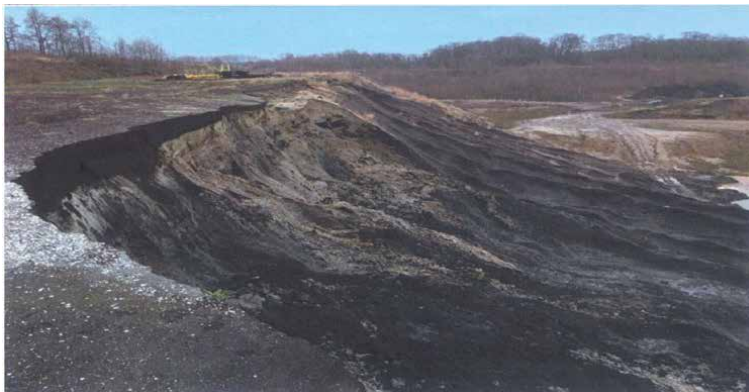
Figure 18. Smoothing of the slope.
