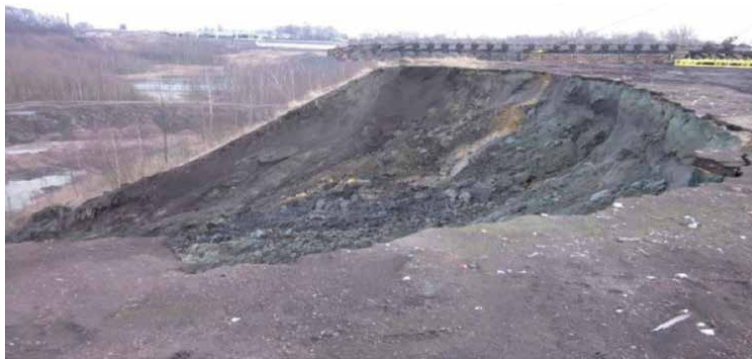
Figure 8. Photo of the unstable zone after the instability of the slope (as adapted from Peiffer (2016) [5]).
