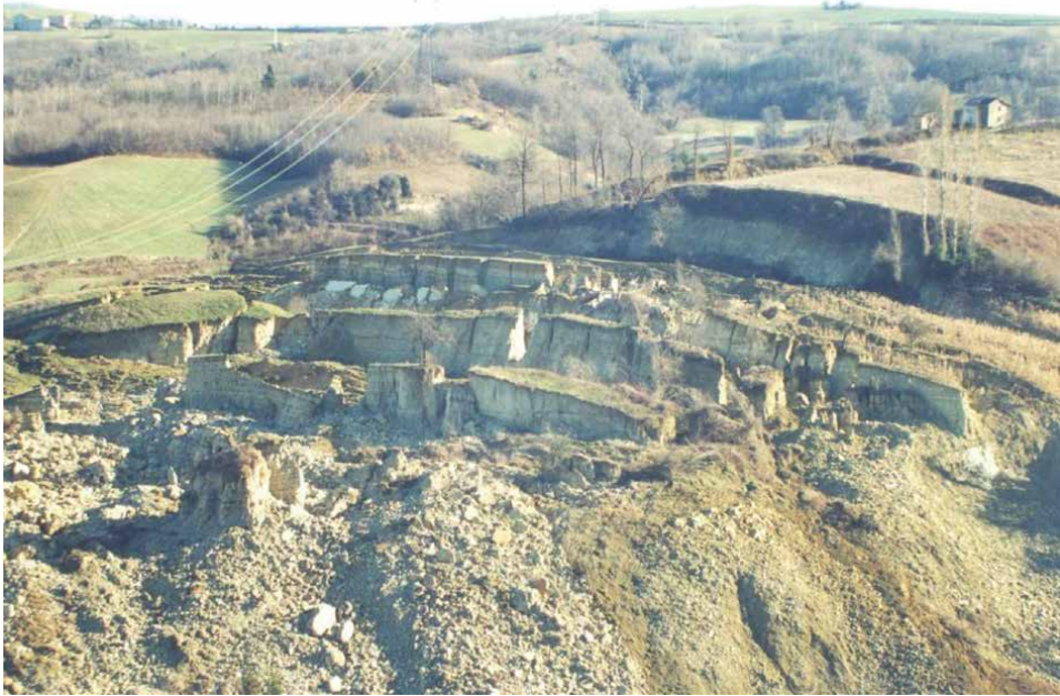
Figure 9. Murazzano Cascina Fascinea farmhouse, one of the most evident landslides of the 1994 event with an area of about 7.4 ha. The clods detached and moved for over 80 m had a height of 8–10 m.
