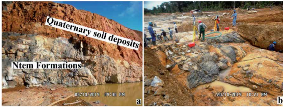
Figure 2. (a) Quaternary soil deposits underlain by Ntem formations that represent two geological units found in the whole dam site and (b) fractured and slightly weathered rock mass.
