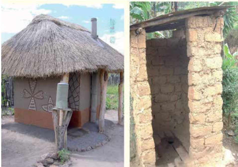
Figure 2. Left: Subsidized ventilated improved pit latrine (VIP) in a CHC home in Zimbabwe with lined pit, concrete slab and vent pipe - a fly trap which eliminates smell and a hand washing facility. Right: An unsubsidized traditional pit latrine in Rwanda, unlined and open pit, log floor giving open access for flies. Photographs courtesy of J. Waterkeyn.
