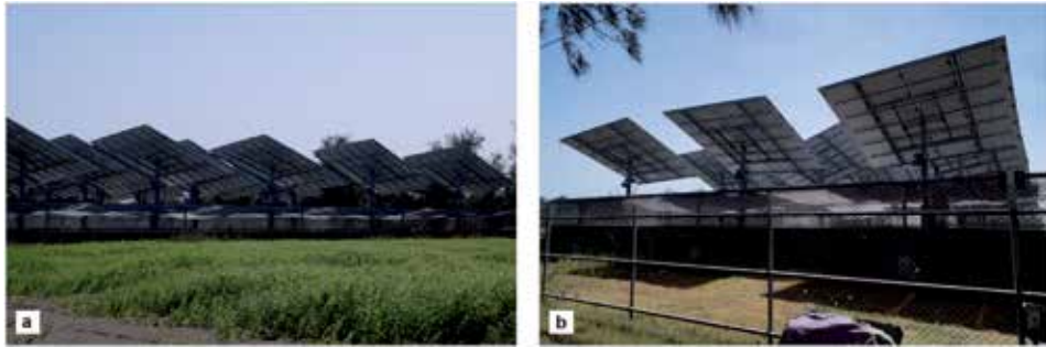
Figure 3. (a-b): Photovoltaic arrays in central Yunlin County with solar trackers to allow for higher efficiency by tracking the direct sunlight beam. Less dense module spacing allow for mixed-land use if feasible.
