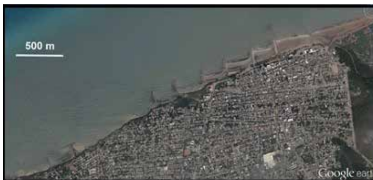
Figure 18. Aerial view of the Riohacha shoreline. Note the large amount of sand accumulation at the east-most three groins and little to no sand accumulation at the rest of the groins and erosion further downdrift.
