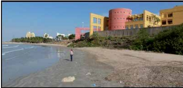
Figure 20. Severe beach erosion downdrift of the Riohacha groin field, exposing a crucial infrastructure to direct wave attack.
