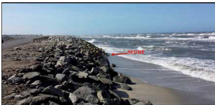
Figure 17. Severe beach erosion at 19 km site threatening a major highway. The recently installed riprap is experiencing toe scour due to continued erosion.
