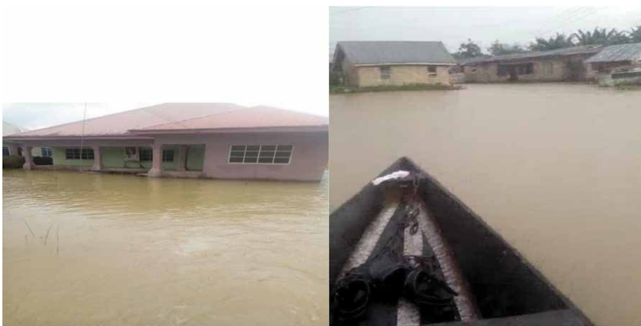
Figure 8. Flooded streets and abandoned houses where residents have migrated.
