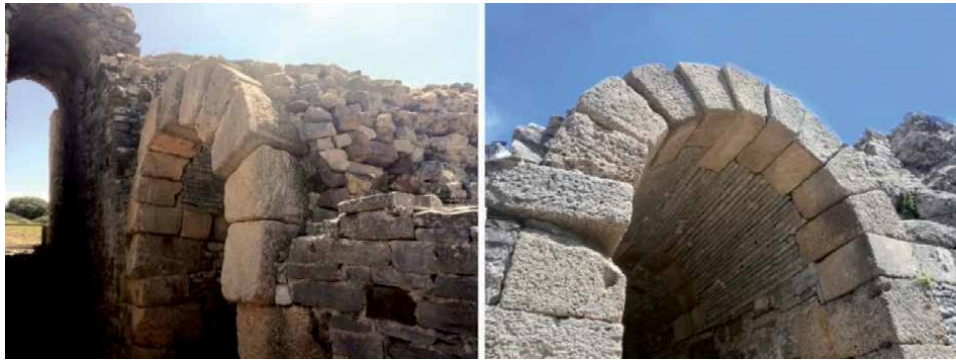
Figure 15. Baelo Claudia, roman ruins (theatre): bowing of a vomitorium wall (left) and expulsion of voussoirs near the parascenium (right), which show a tensile stress in the direction of the slope. Source: J A Aparicio.
