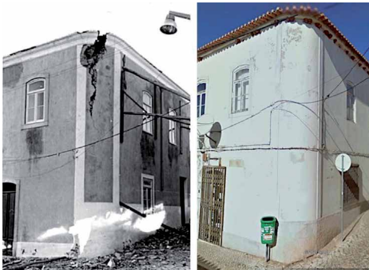
Figure 5. Vila do Bispo, building of class A with damage of grade 3 due to loss of connection between load-bearing walls and corner failure (left). This two-story house was repaired and is currently in use (right). Sources: IPMA/Google Earth.
