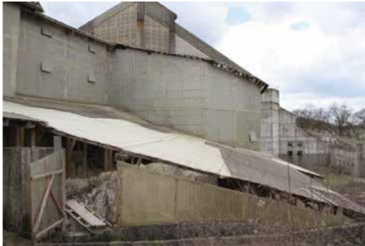
Figure 2. Provisional protection structure.
