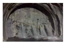
**Figure 7.** Water inrush after tunnel excavation.
