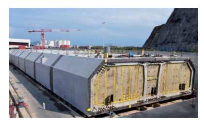
Figure 10. Photo of immersion joint of tunnel element in HZMB Island-tunnel project.
