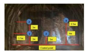
**Figure 5.** *Position of the lead drilling hole.*
