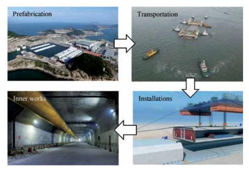
Figure 2. Construction works of the immersed tunnel in HZMB Island-tunnel project.
