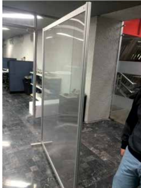
Figure 5. Transparent acrylic mounted on an aluminum base.
