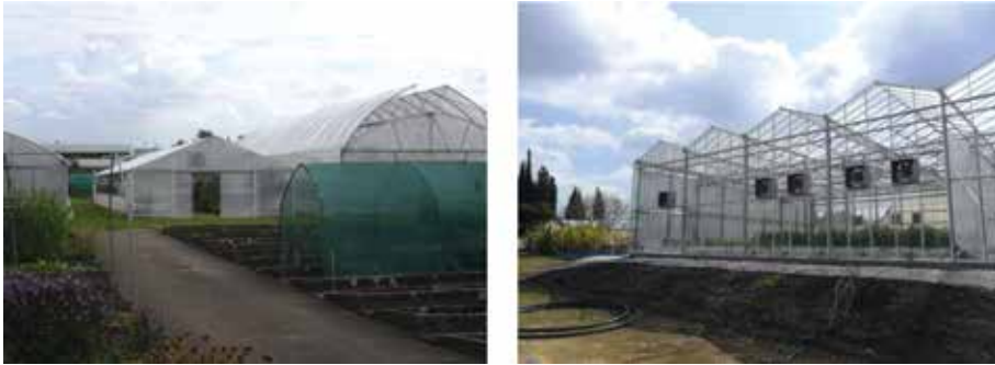
Figure 1. Natural and mechanical climate control in greenhouses.
