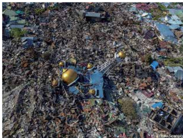
Figure 12. Indonesia Sulawesi Island earthquake and tsunami damage (after Reuters/Aflo).
