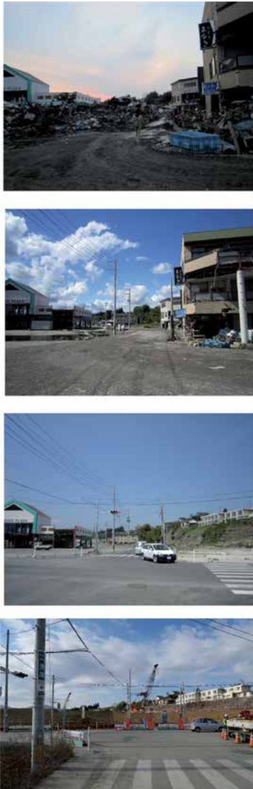
Figure 11. Restoration of Kesennuma City of Miyagi Prefecture in Tohoku district during 4 years (after associate professor M. Sakamoto of Nagoya University).
