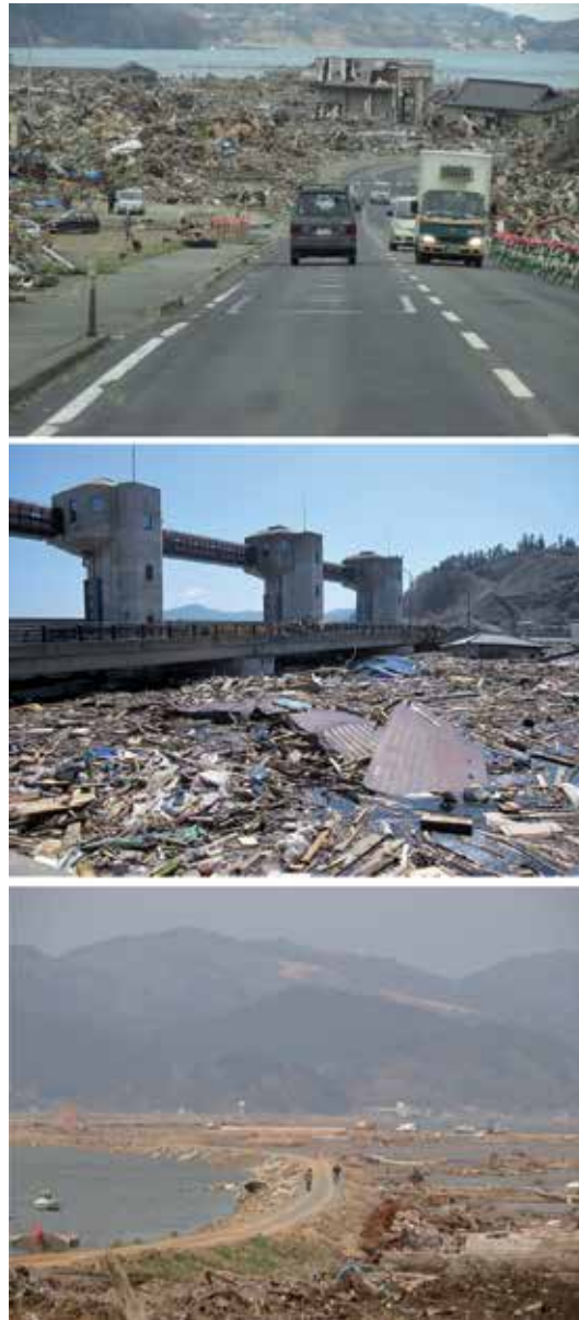
Figure 3. Damages by 2011 East Japan earthquake. (Above) Damaged Onagawa city in Miyagi Prefecture (after associate professor Sakamoto of Nagoya University). (Middle) Damaged Otsuchi city in Iwate Prefecture (after Mr. Satoshi Nagao). (Below) Damaged Kitakami River in Iwate Prefecture (after associate professor Sakamoto of Nagoya University).
