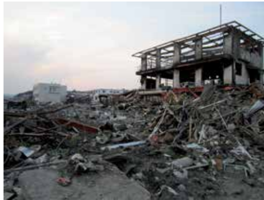
Figure 1. Damages by 2011 East Japan earthquake (after associate professor Sakamoto of Nagoya University).
