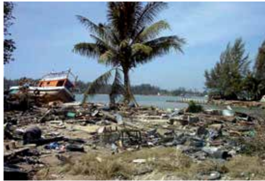
Figure 2. Damage by 2004 Sumatra tsunamis (after the Ministry of Foreign Affairs in Japan).
