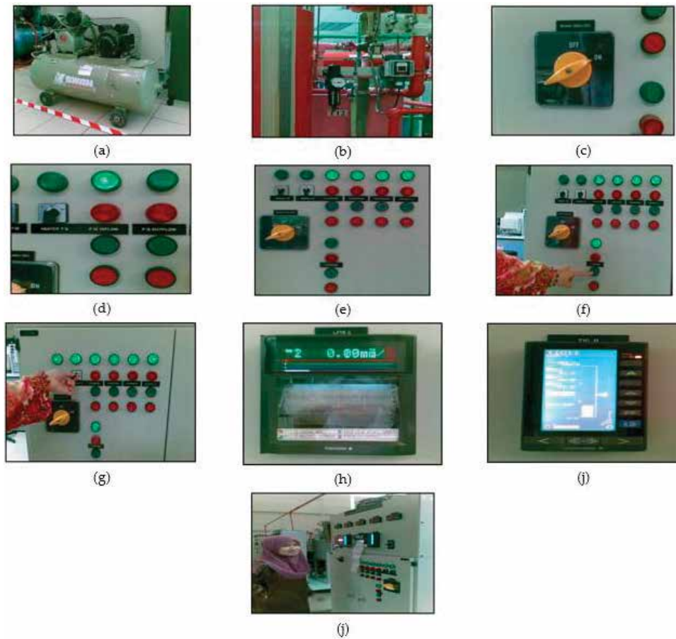
Figure 4. (a) Start on compressor. (b) Supply AIS. (c) On main switch (415V/3P). (d) On P12 inflow and P11 outflow. (e) P13 and P14 product. (f) On P15 mixing. (g) On heater T12 and T11. (h) Check recorder LFTR1. (i) Temperature controller TIC. (j) Output graph.
