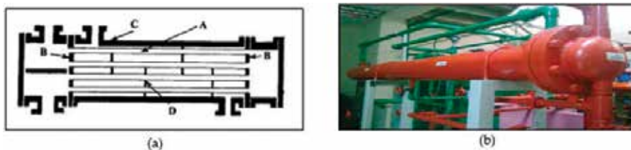
Figure 1. (a) Diagram of a typical shell and tube heat exchanger. (b) The heat exchanger QAD BDT921.
