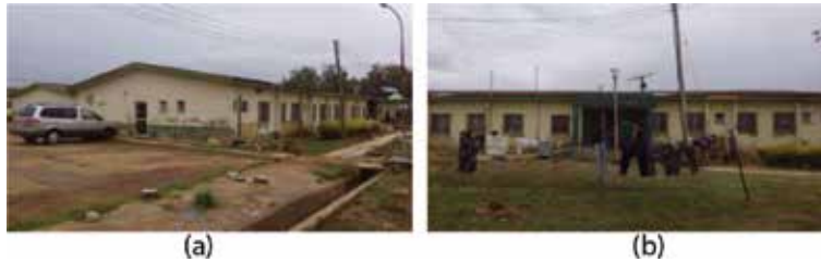
Figure 5. Exterior views of Specialist Hospital ward—(a) northeast view, (b) southeast view.
