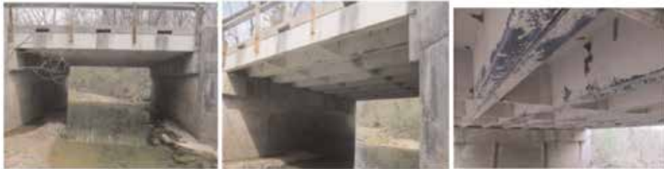
Figure 4. Creasy Springs Road bridge.
