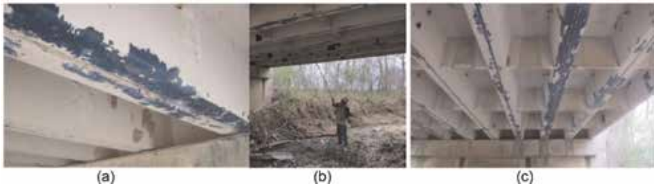
Figure 7. Coats Lane bridge—testing channel beams. (a) Second beam, first channel, (b) impact testing, (c) beams 6–8.
