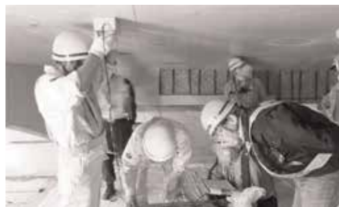
Figure 12. Field experiments of checking the railway bridge.
