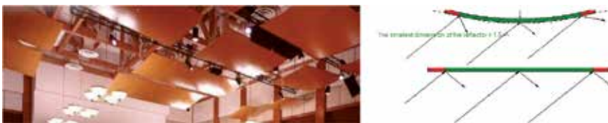
Figure 10. Reflectors appearance in the interiors on the left and the difference of dimensions between the flat reflectors in comparison to the convex reflectors on the right.
