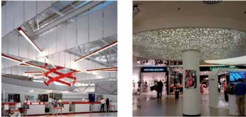
Figure 8. Public announcement (main corridor in a mall where absorber patterns in the ceiling on the right and principal hall in airport where absorber baffles on the left).
