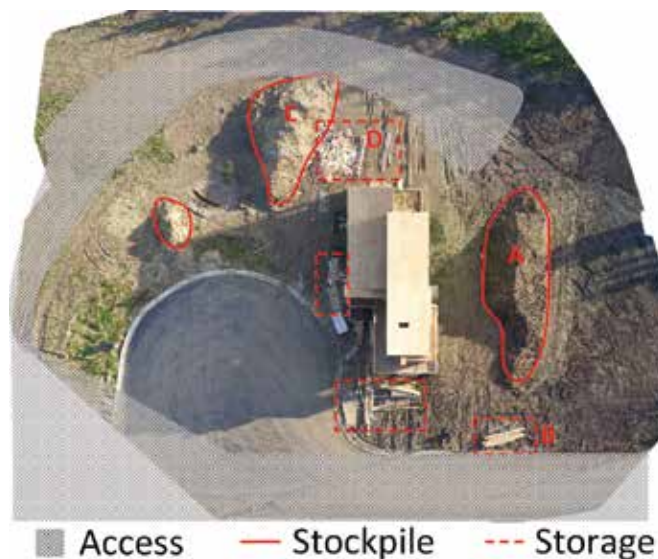
Figure 4. Qualitative constraints identification in GoogleEarthWork: geo-relationship between accesses, stockpiles, storage area, and the building identified from high-resolution panoramic images stitched from aerial photos.
