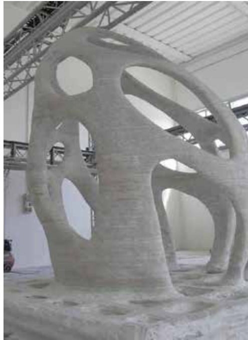
Figure 10. D-shape printed monolith ( https://tinyurl.com/y8c87o6z ).
