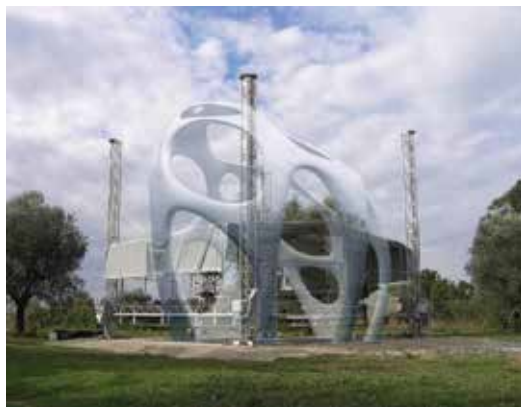
Figure 9. D-shape printed monolith ( https://tinyurl.com/ybdf339t ).
