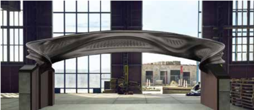
Figure 13. Robotically printed metal bridge ( https://tinyurl.com/yanqvhv9 ).
