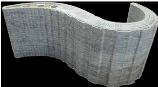
Figure 11. Concrete printing ( https://tinyurl.com/ydd8lmsa ).
